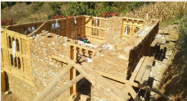
Figure 17 Kelzang's new house under construction
