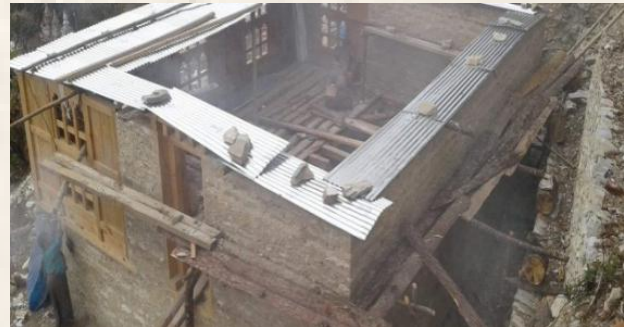
Figure 47 Tshering house nearing completion
