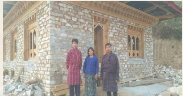
Figure 38 Ugyen & family in front of their new house
