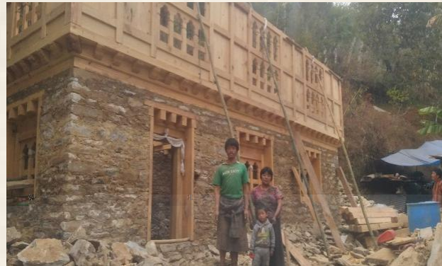
Figure 41 Sangay's new house under construction
