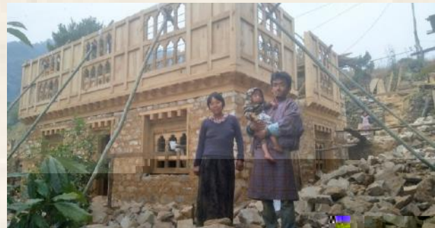
Figure 43 Leki & family at the construction of their new house
