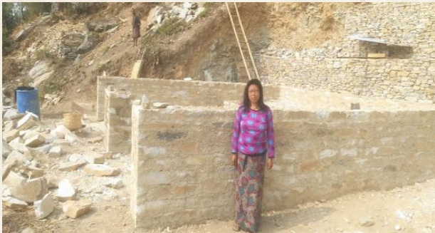
Figure 46 Tshering at her house construction
