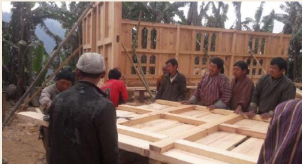
Figure 55 Bumpa's house under construction
